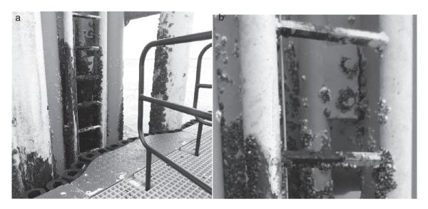
Fig. 2a & 2b. Examples of the external ladder on a turbine. NB. Figure 2a depicts a vessel up against an external ladder.
