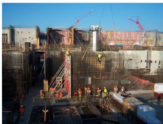
Figure 1. The new facility walls and levels in full construction phase.
