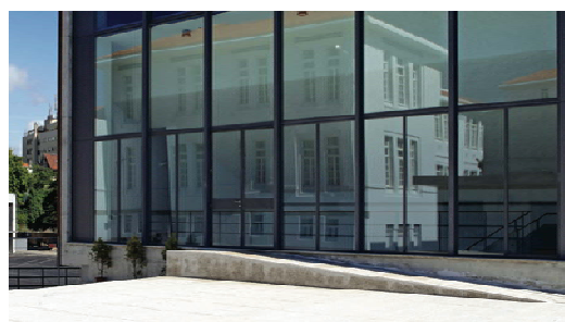
Figure 2 - Building access ramp. High School Rodrigues de Freitas. Project: Manuel Fernandes de Sá, architect.
