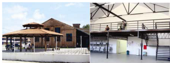
Fig. 02: Facade and lobby of the Classes Central
