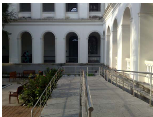
Image 21 Ramp of the Hospital Pedro II
