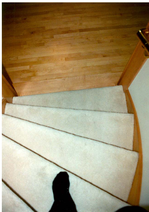
Fig. 5. As seen from above the stairs and the lower landing are quite apparent. The bottom tread is not conspicuous. (The photographer's foot, however, is.)
