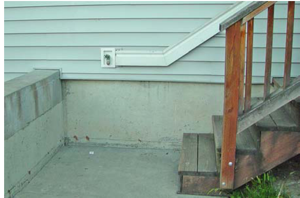
Fig. 2. She was not aware the handrail on her left ended before the bottom landing.
