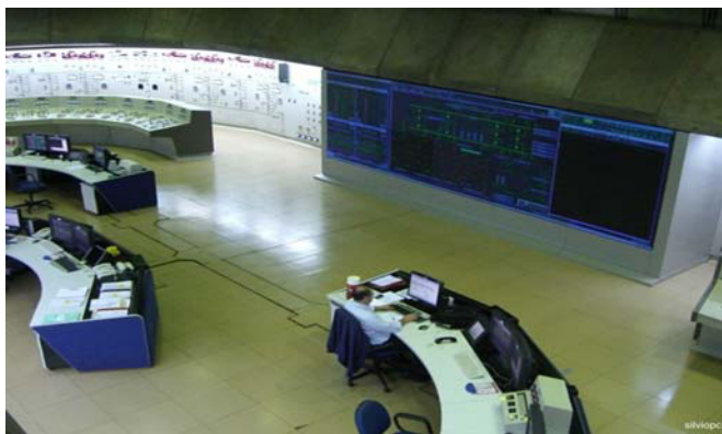
Figure 3 The typical Electric Power control Centers
