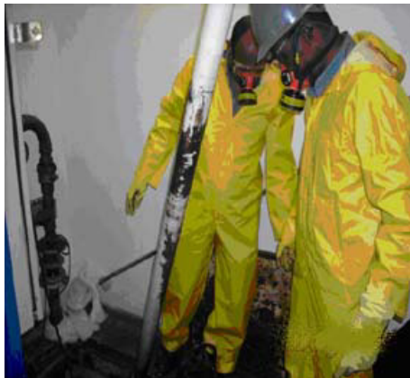
Figure 5 – Tubing infected of waste – For the task, the overall maintenance and use PPE Tayvec (waterproof fabric), half-face mask, PVC gloves, but even with the use of PPE they are exposed to biological and ergonomic risks.
