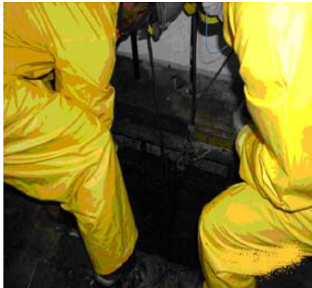
Figure 11 – Sequence of the task of lifting the pump in the tank.
