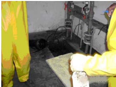
Figure 6 – Use of PPE (coveralls Tayvec - waterproof fabric) semi-facial mask, PVC gloves.
