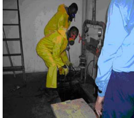
Figure 8 – Sequence of the task of lifting the pump in the tank.
