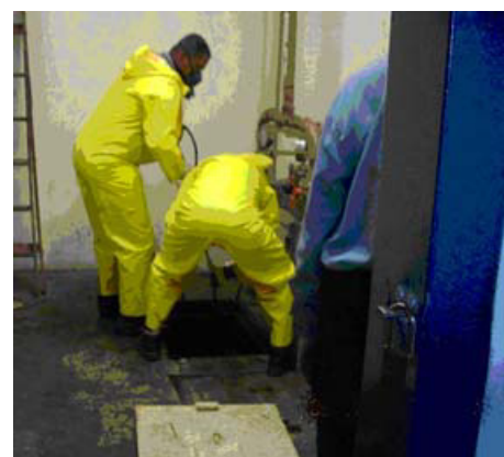
Figure 10 – Sequence of the task of lifting the pump in the tank.
