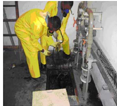
Figure 9 – Sequence of the task of lifting the pump in the tank.
