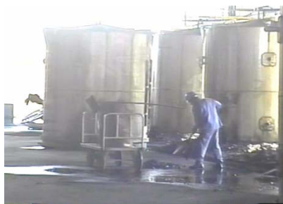
Figure 5 – Carbonization Place Cleanup
