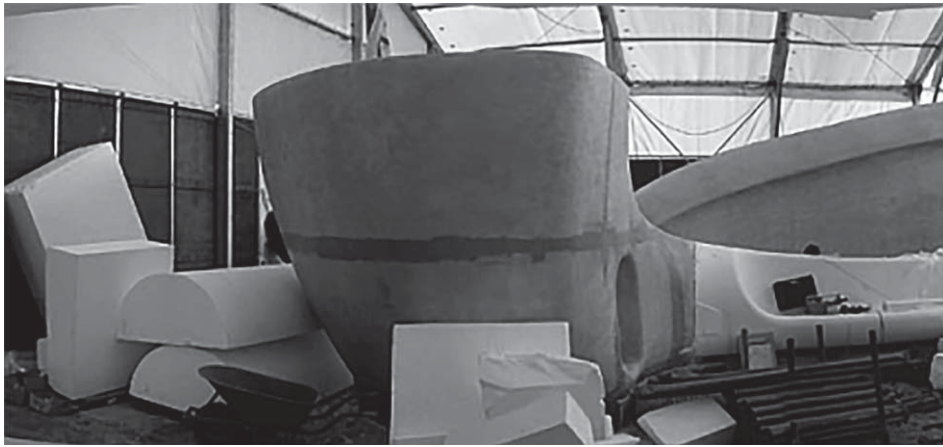
Fig. 4. Moulds of polystyrene foam for Bus Station in Hoofddorp, the Netherlands (2003).
