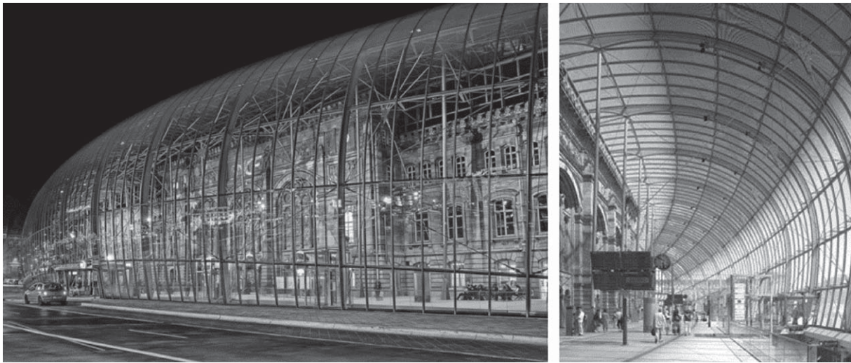
Fig. 3. Example for cold bent glass by assembling (Fildhuth, 2014).
