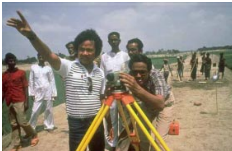
Filipino volunteers work on road construction in Bangladesh (UN Photo)
