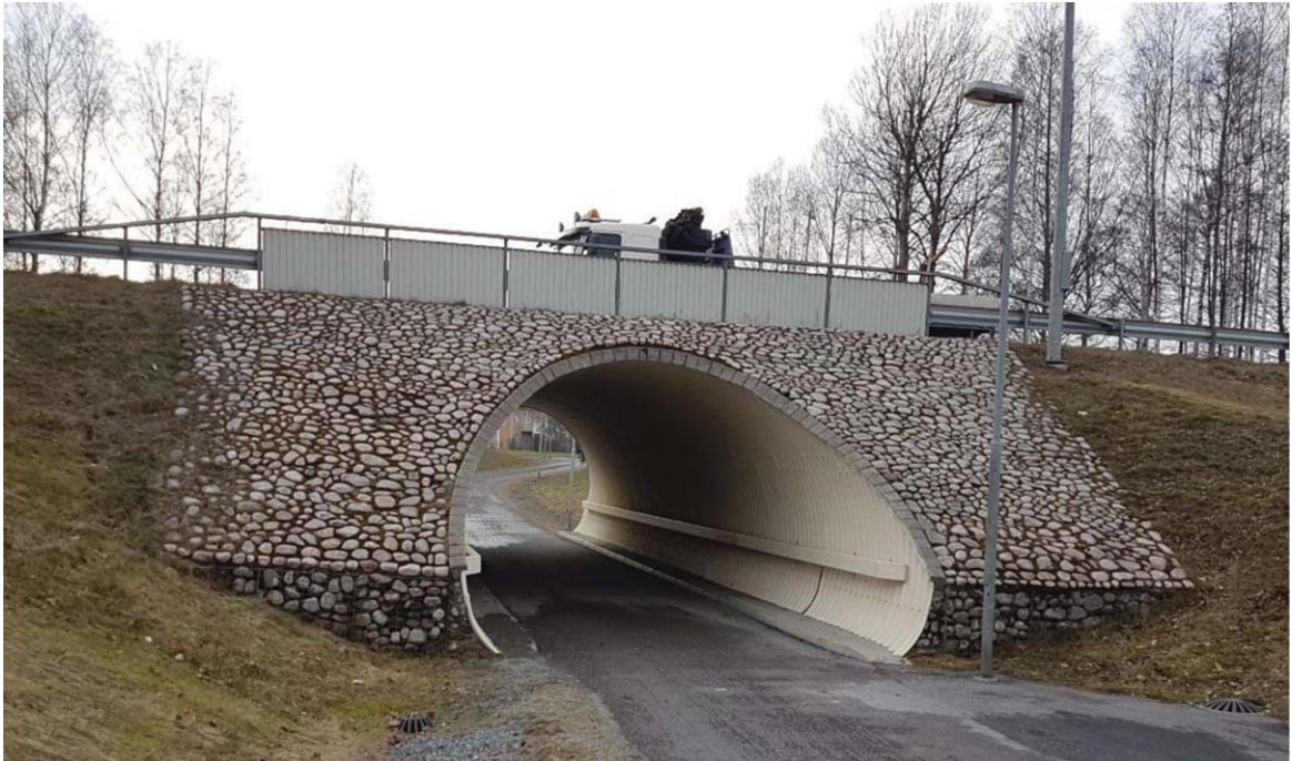
Fig. 1. Soil-Steel Composite Bridge over a pedestrian walkway in Lidköping, Sweden.
