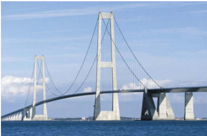
Fig. 26. The Great Belt Link's suspension bridge and one of its piers selected for testing for service life. The pier was constructed using plywood form kept on for 2-3 days before stripping. LOK-TEST performed met the requirements.
