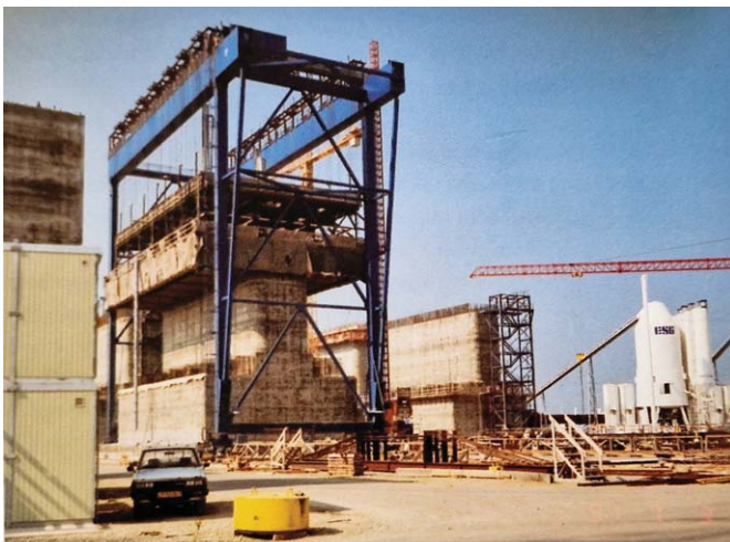
Fig. 23. Steel slipform used for the caissons (left), and CAPO-Testing (right).
