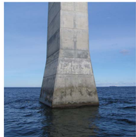
Fig. 26. The Great Belt Link's suspension bridge and one of its piers selected for testing for service life. The pier was constructed using plywood form kept on for 2-3 days before stripping. LOK-TEST performed met the requirements.
