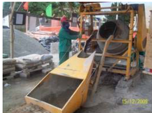
Figure 3: Mixer on site "b"
