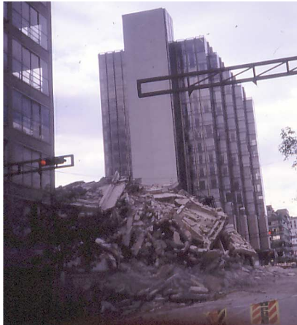
Fig. 1. Impact of earthquake on Access de Mexico Office Building. (Colors are visible in the online version of the article; http://dx.doi.org/10.3233/ISU-140726 .)
