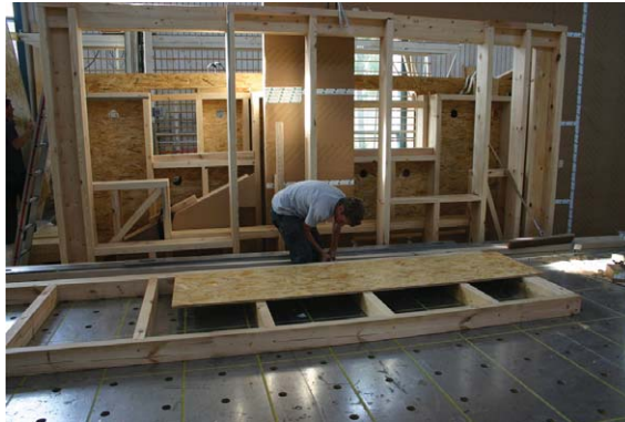
Fig. 1. Wall assembly at the Berchtold Holzbau factory in Voralberg.
